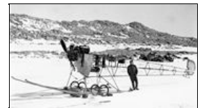
Mawson's Huts Foundation
